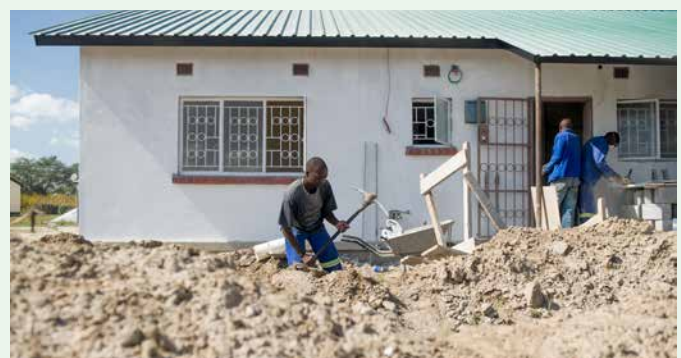
▲ A new staff house under construction. ob
