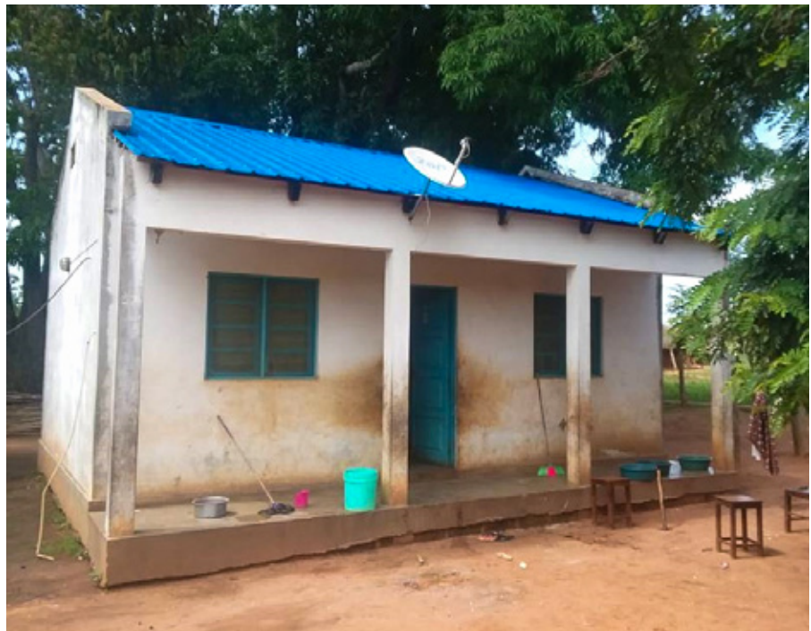
▲ SolidarMed repairing the roof on this staff house at the Ncumpe health care centre in Namuno, Mozambique. sm
